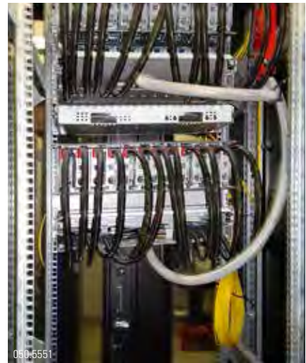
Custom product for the Linxdatacenter in Warsaw: R&M global patch fields.
