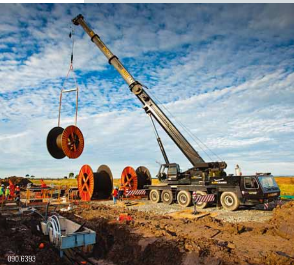
Installation of a section of the 87 km underground power cable, which will supply power to Victoria's new desalination plant
