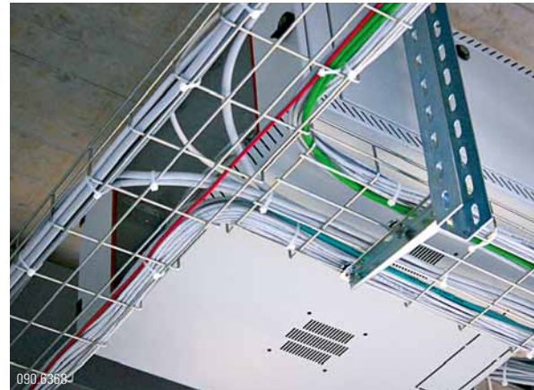
Consolidation point (CP) cabinet installed on the ceiling
