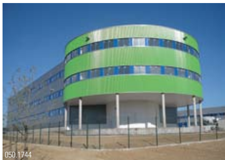
050.1744 The Casbar company HQ: one of Spain's top manufacturers of outdoor cabinets
