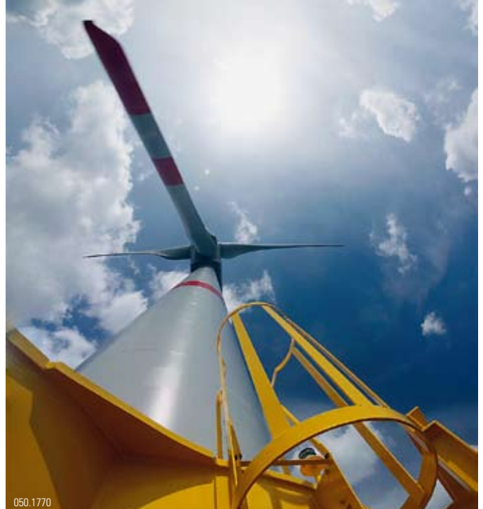
A BARD offshore wind turbine has a total height of about 152 meters; the rotor has a diameter of a good 122 meters. (Source: BARD-Group/Meyer)
