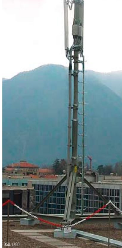
050.1780 Rooftop location for antenna
