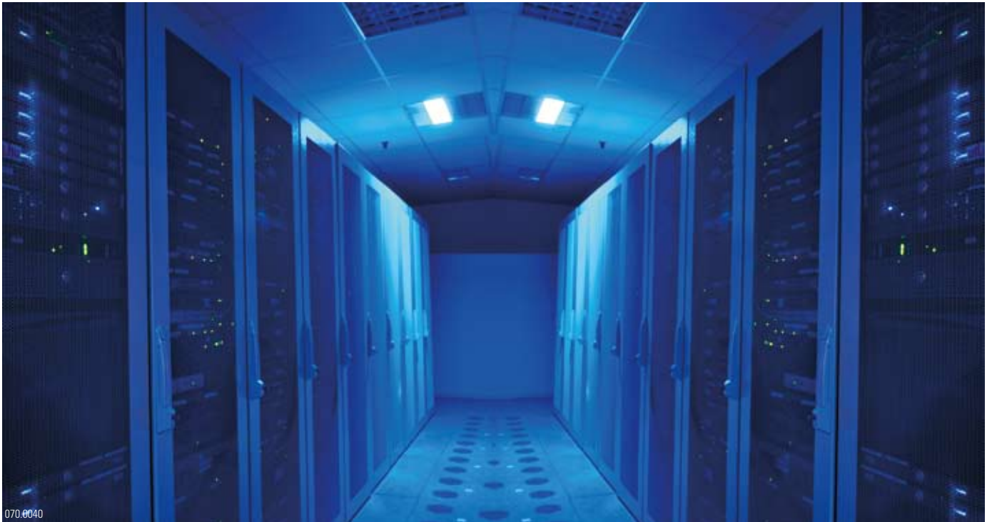
070.0040 New chances but also new challenges – the modern data center is multifaceted and complex yet opens up many possibilities.
