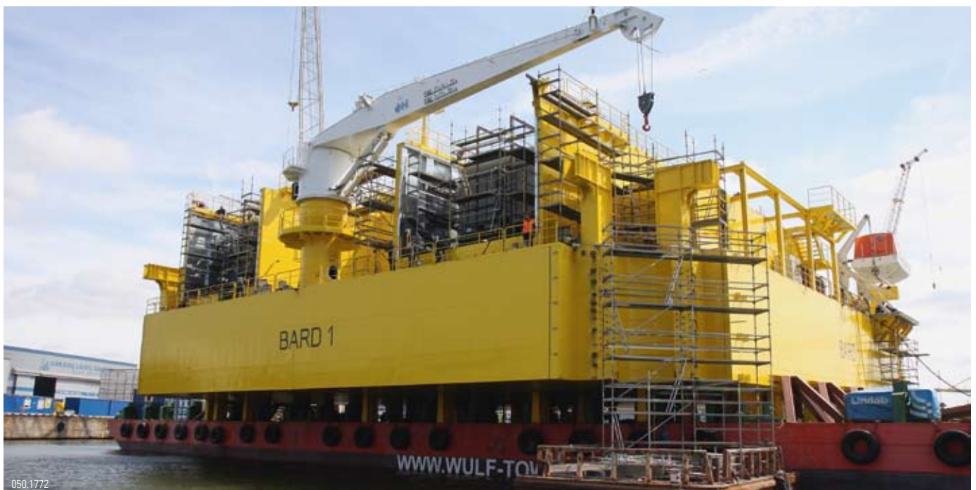
The top site for the BARD residential and transformer platform during the construction phase at WSY dockyard in Klaipeda, Lithuania: On completion, it will be installed in the BARD Offshore 1 wind park. (Source: BARD-Group)
