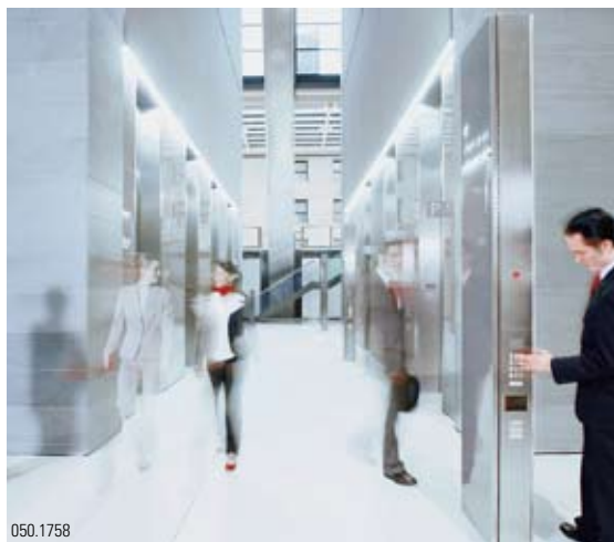
Elevator lobby showing Schindler's Miconic 10 destination control system: It calculates which elevator will reach which floor fastest, and directs passengers to the car taking the most direct route to their floor. The desired floor is punched in before the passenger enters the elevator.
