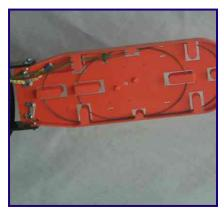
**20** Splice fibres in accordance with standard jointing practise, and neatly coil away fibres into the fibre tray.
