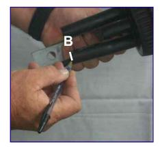
Mark the cable B level with the bottom of the heatshrinkable sleeve.
