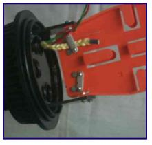
Pull back the cable and pass the GRP strength member and aramid yarn between the GRP link and fibre tray.
