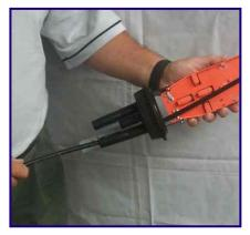
Pass cable through open cable entry port, leaving sufficient length of cable for splicing ±1.5M.
